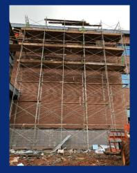
Brick nearing completion at Elevation K (exterior of gang restrooms)
